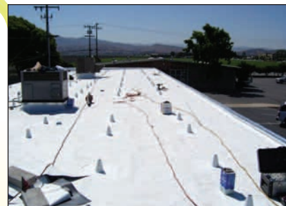
Custom Solar Flashings for Single-Ply Systems
